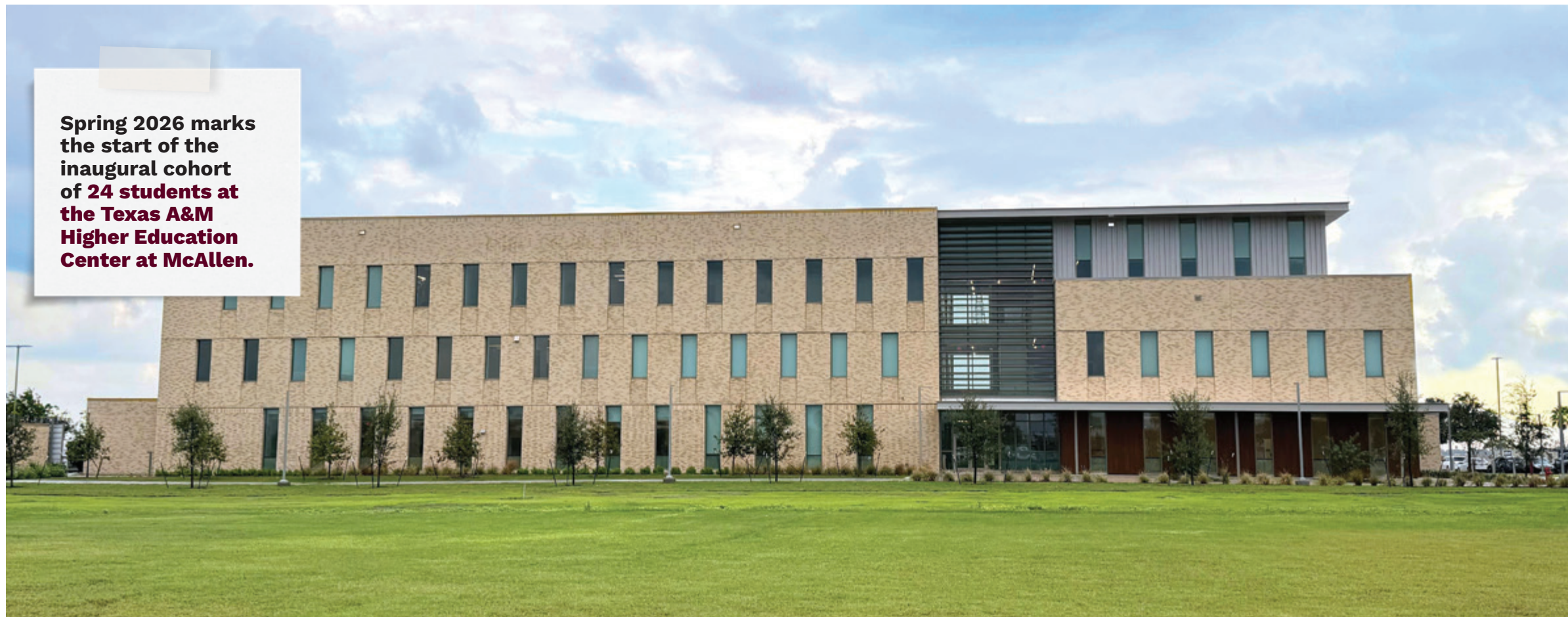
The Nursing Education and Research Building at the Texas A&M Higher Education Center at McAllen.
